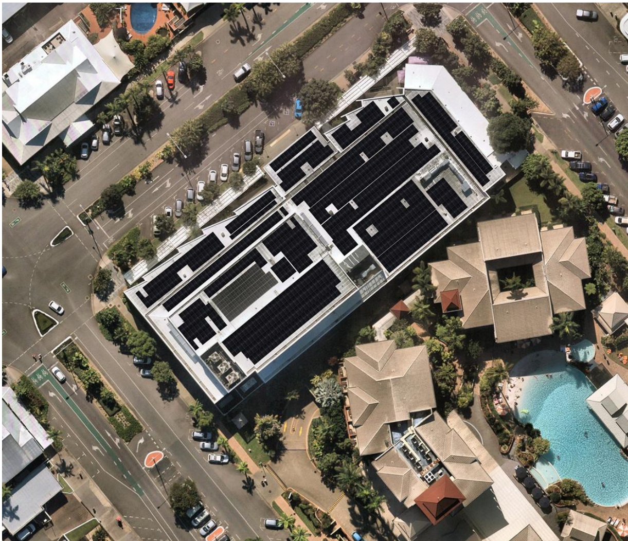
Image: The Cairns Aquarium 1 acre inner city rooftop transformed into a microgrid with almost 700 High efficiency solar panels.
